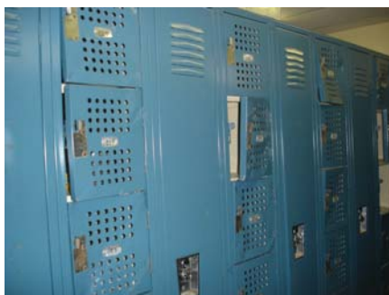
Locker room replacement
