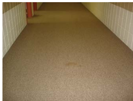
Replace original carpeting
