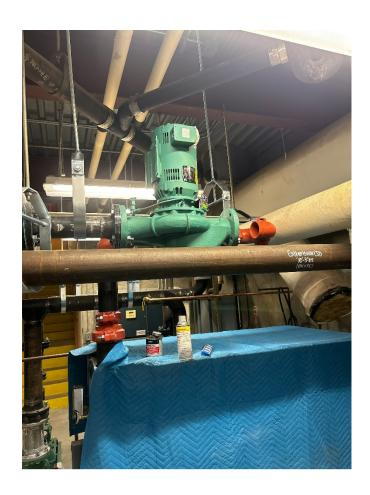
Friday 6/18/24 – Installation of Boiler Circulating Pumps and piping in progress.
