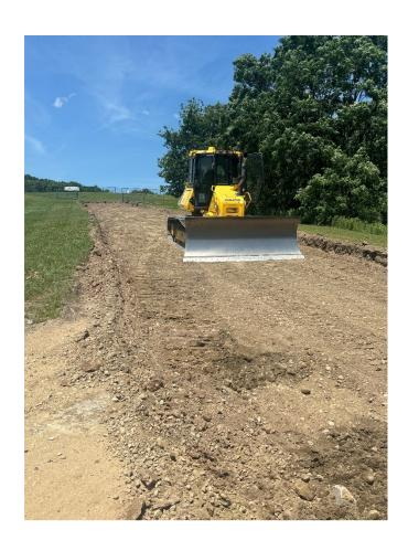
Wednesday 7/03/24 – Upper Drive - Milling of asphalt completed. Removal of existing subbase and placement of new subbase material to follow.
