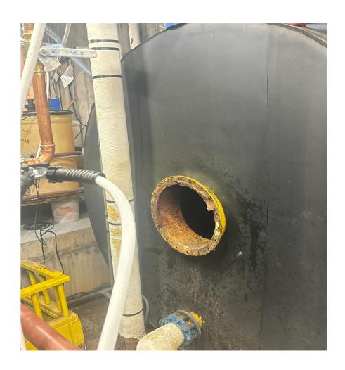
Wednesday 7/03/24: Main Building – Boiler Room – Draining of water storage tank, and removal of access port cover completed. Cleaning and relining of tank to begin Monday 7/08.
