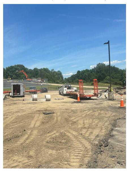
Wednesday 7/03/24 - Main Drive - Milling of asphalt completed. Removal of existing subbase and placement of new subbase material to follow.
