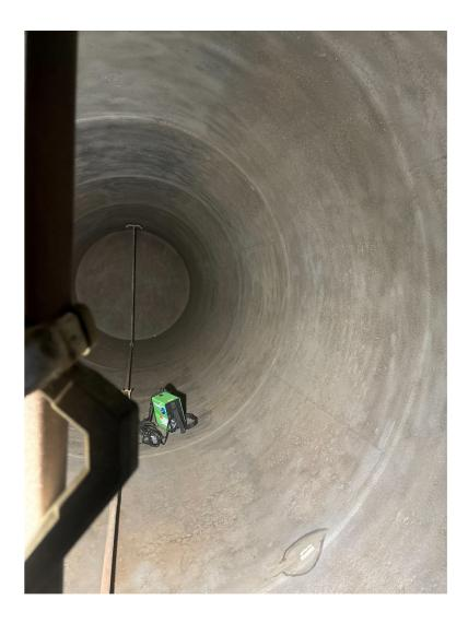
Tuesday 7/09/24 – Interior of Main Building Water Storage Tank: Storage Tank cleaned, sandblasted and lining applied 7/09.–
