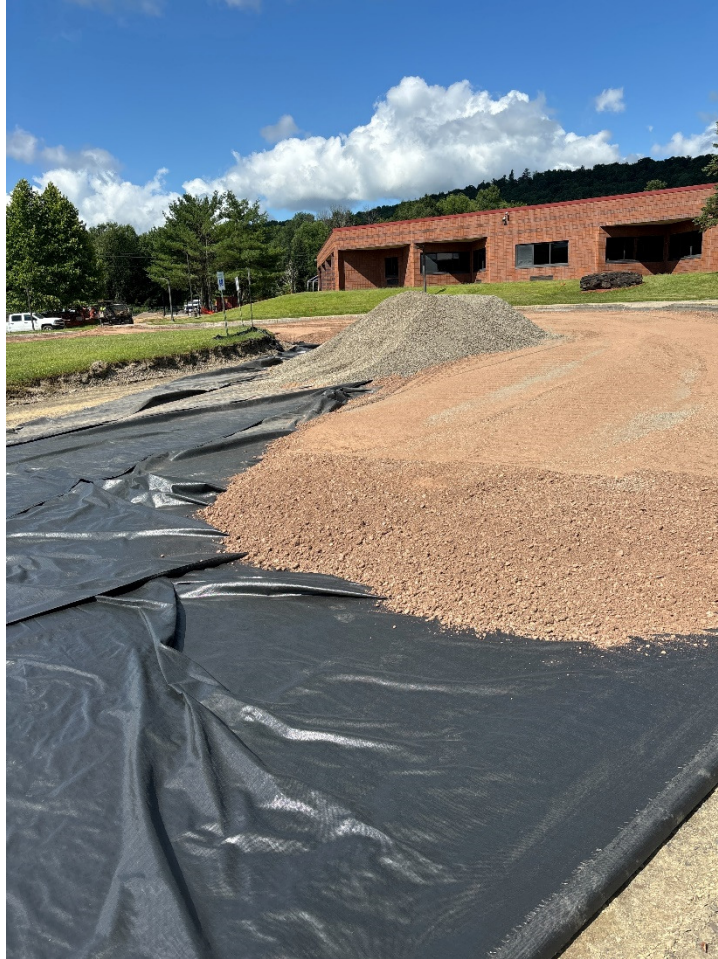
Friday 7/19/24: Bus loop – Placement of Fabric and subbase materials in progress.
