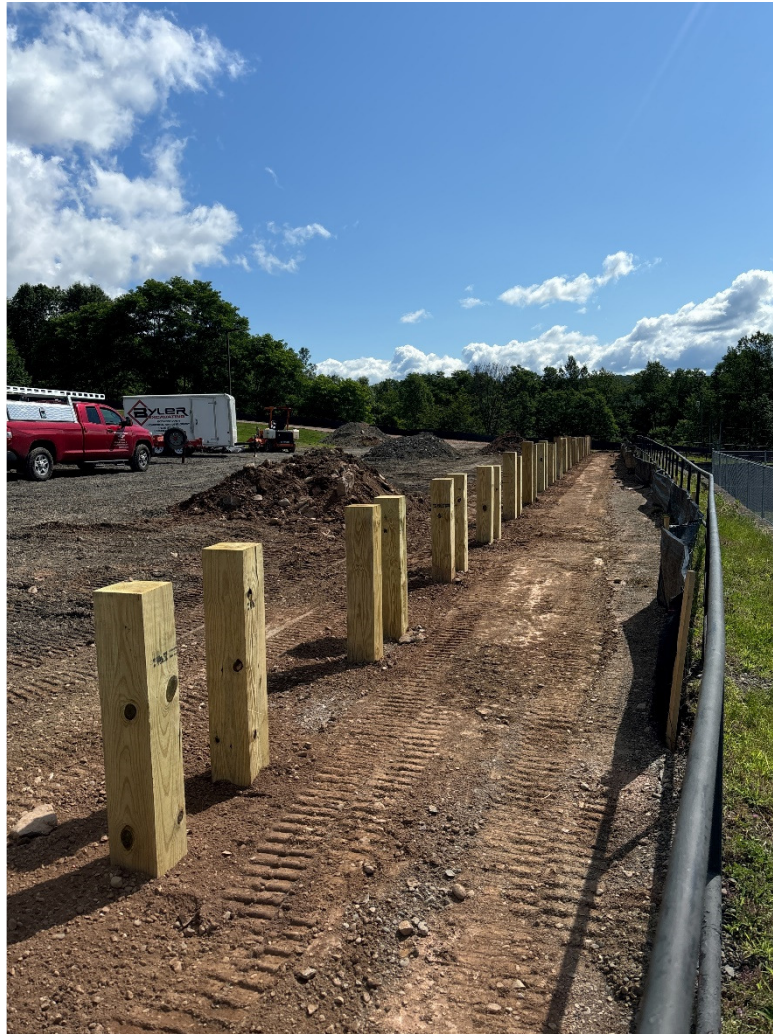
Friday 7/19/24 – Upper Parking Area – Installation of guardrail posts in progress.
