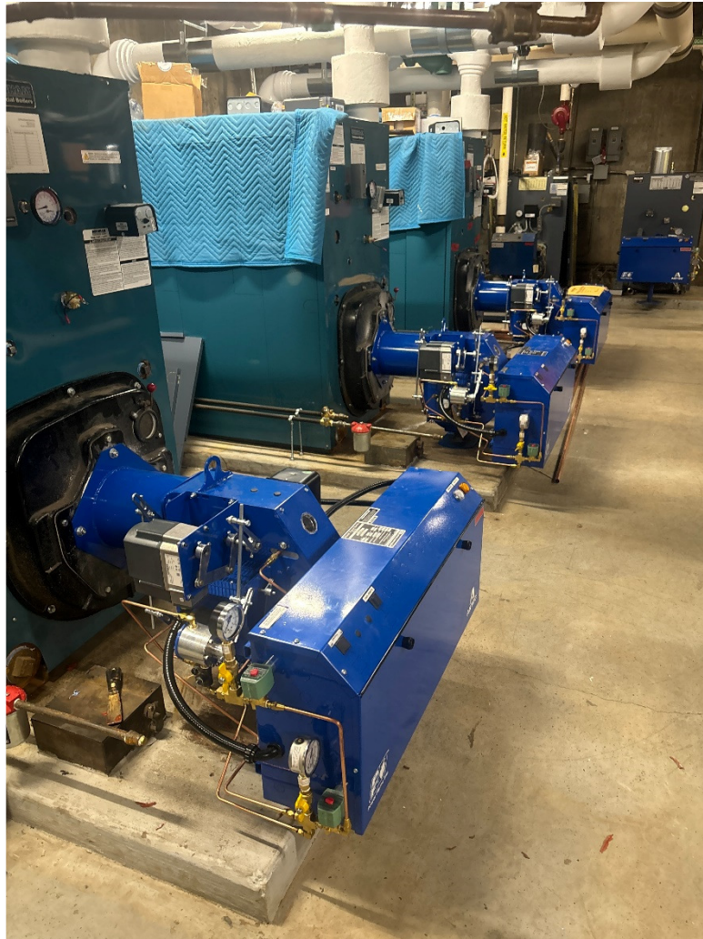
Friday 7/26/24 – Boiler Room – Installation of burners for new boilers in progress.
