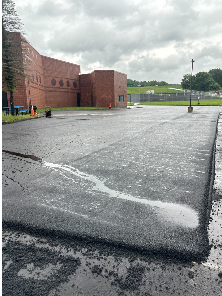
Friday 8/09/24: Main Parking Area "D"- Application of Asphalt Paving Top Course in progress.
