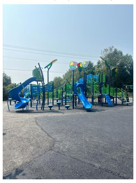
Friday 8/16/24: Playground – Main Play Structure pictured. Installation of play structures and asphalt paving completed. Installation of rubber tile safety surfacing to follow.
