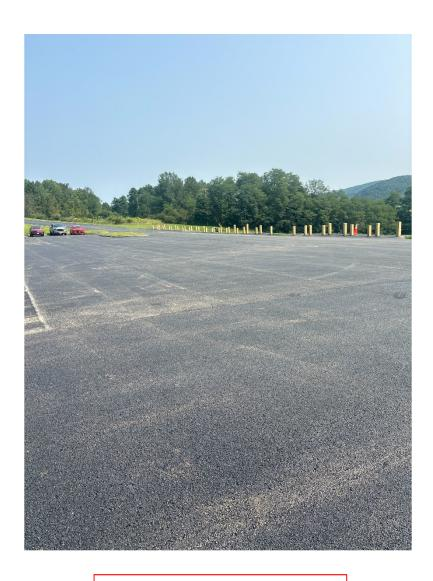
Friday 8/16/24 – Main Lot-Application of top asphalt coat completed. Installation of guiderail top rail to be performed next week.
