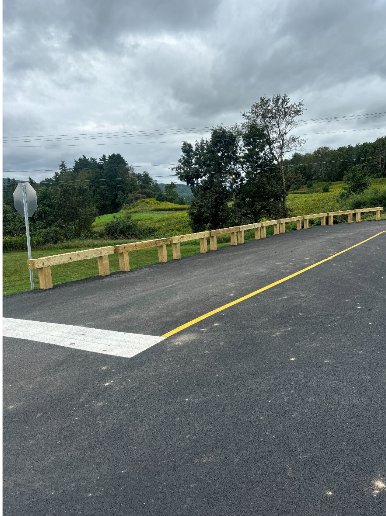
Friday 8/30– Main Drive – Installation of top rail on guiderail completed.
